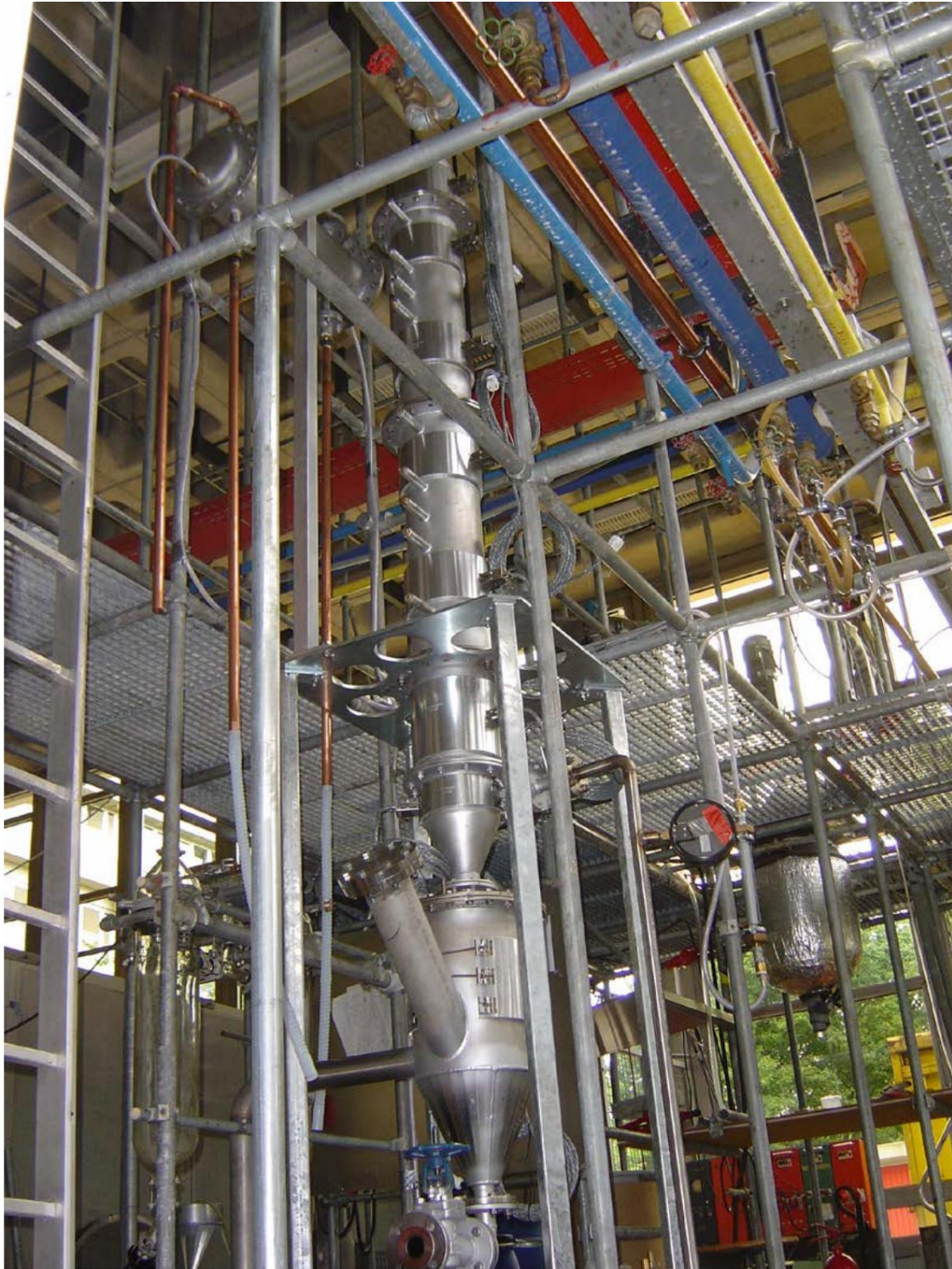
Fig. 15: Semi-continuous 5 kg/h KDV pilot plant under construction
